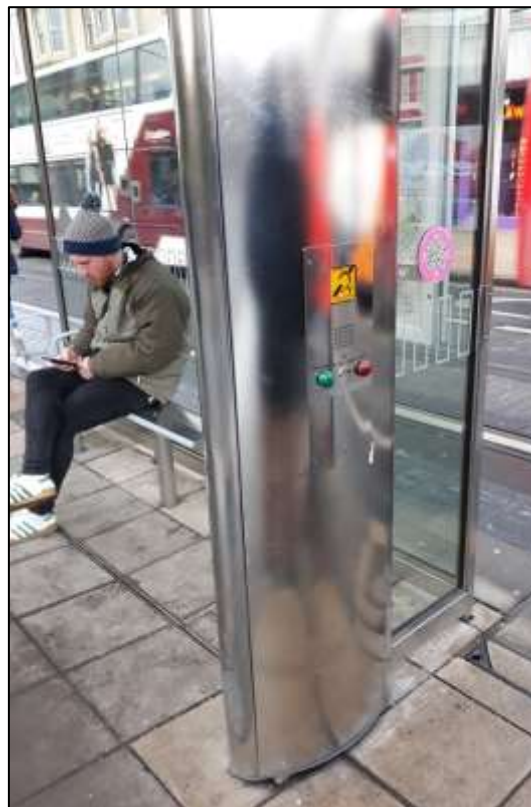
Figure 10: PHP/PECP integrated in shelter (existing design)
