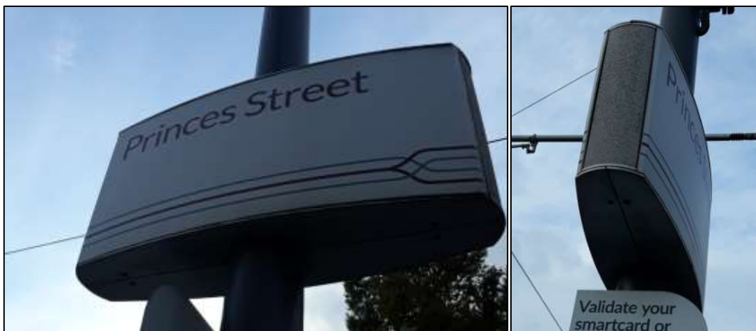
Figure 15: PA speakers integrated in tram stop sign (existing design)
