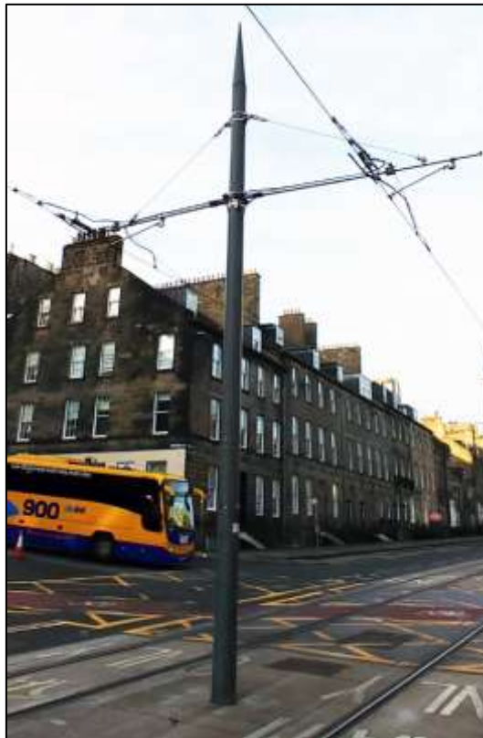
Figure 22: OLE pole (existing design)
