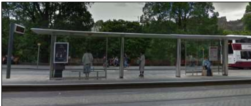
Figure 8: Existing shelter at Princes Street tram stop
