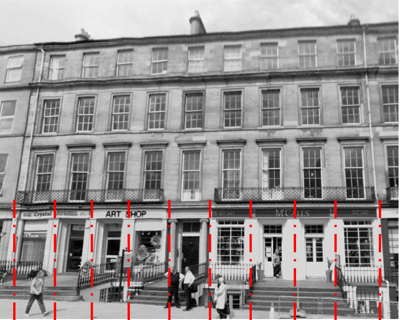
Haddington Place terrace showing ground floor condition of column support every bay
